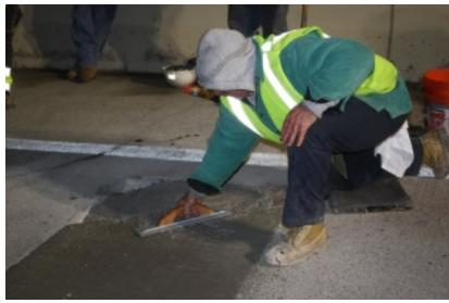
MALP Concrete was trowelled immediately after pouring No curing compound
